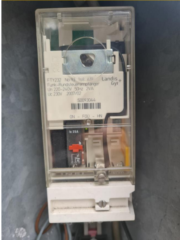
We found a radio-controlled switch for the street light!
