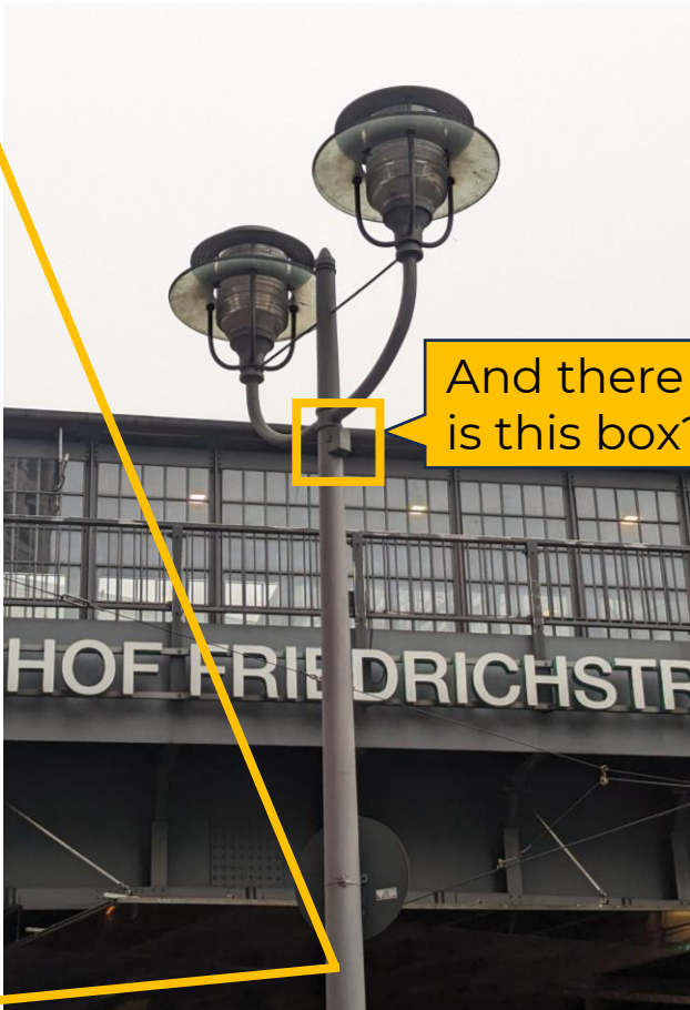
We found a radio-controlled switch for the street light!
