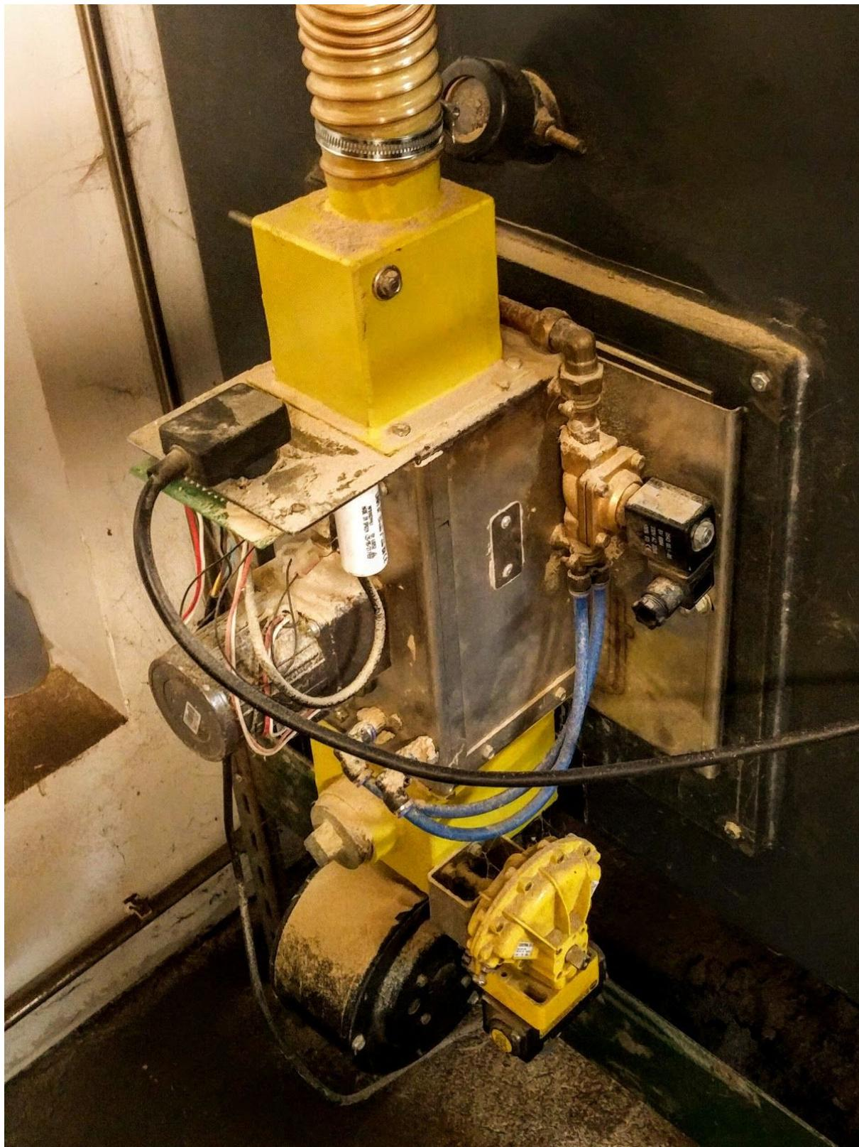
5. Burner controller and MeterLogger device. Note the angled Wifi Antenna protruding under Kamstrup meter
