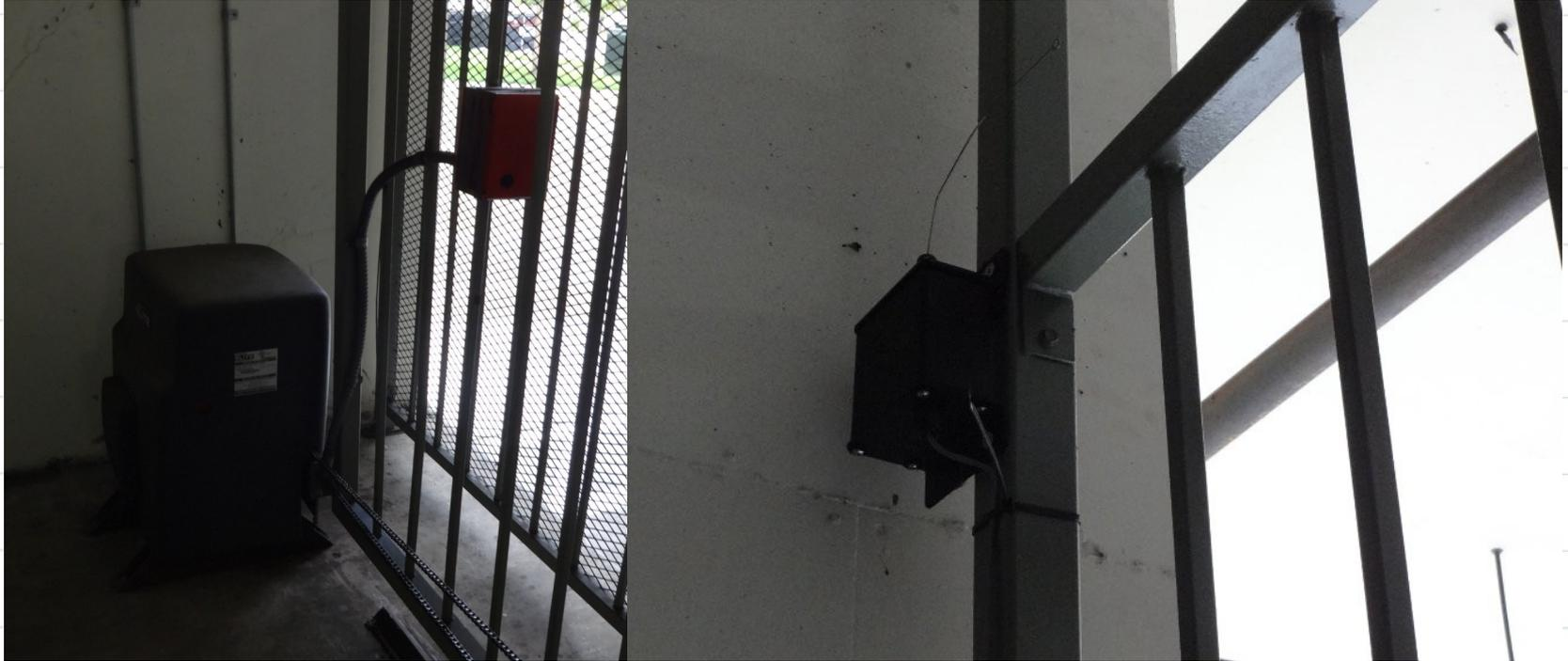
the motor is just triggered by the receiver
