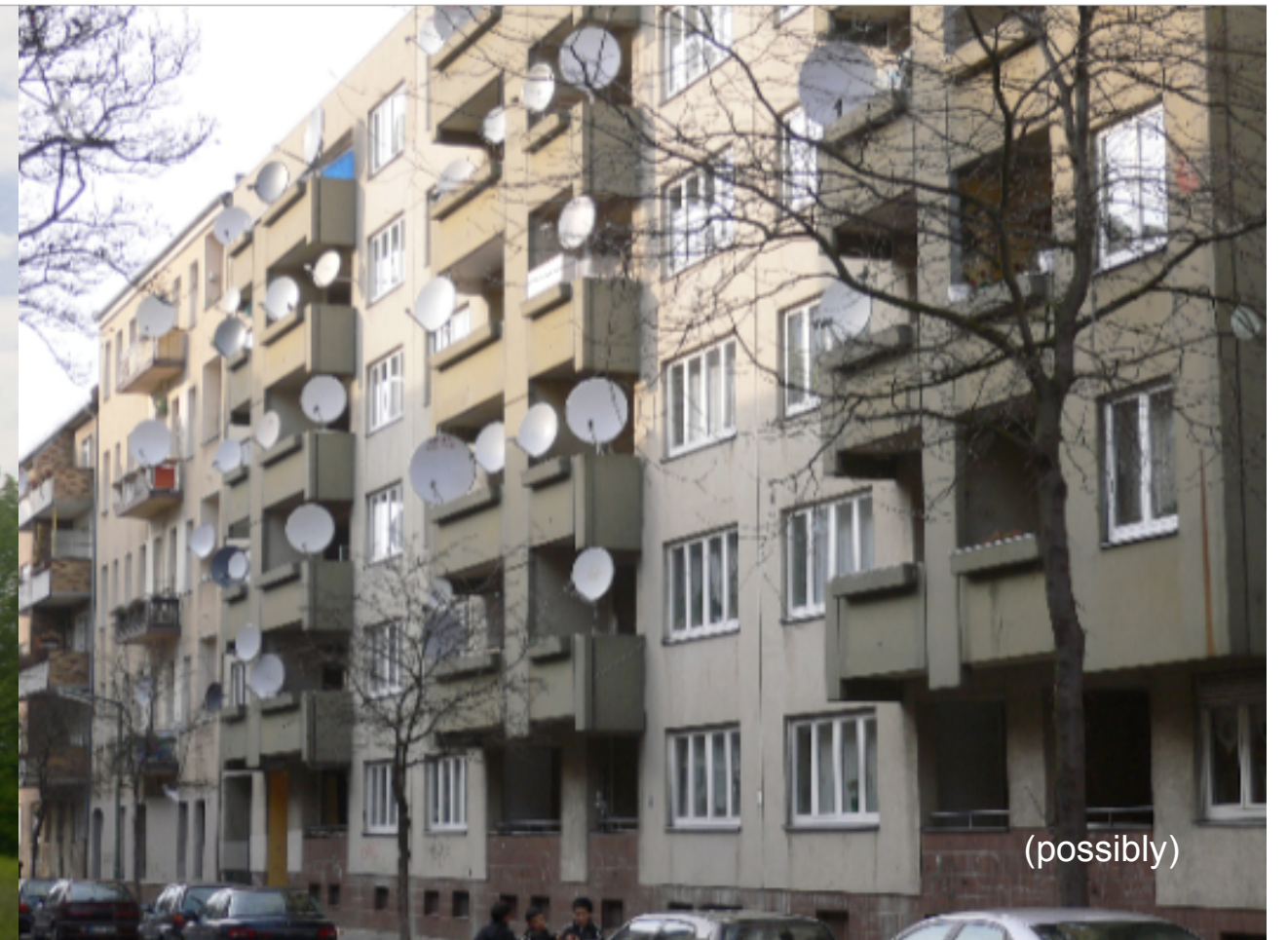
HGG Groundstation, Berlin-Neukölln, Germany
