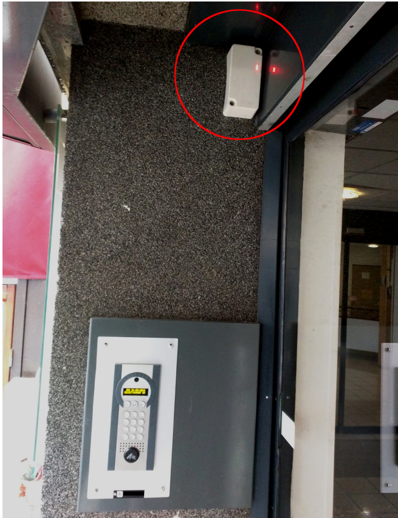
Figure 2: Example of 3G block of an intercom
